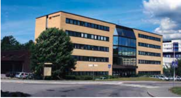
Terco headoffice and factory outside Stockholm, Sweden
